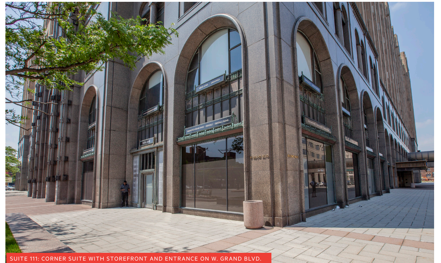
SUITE 111: ENTRANCE INSIDE THE ARCADE FEATURES CHANDELIER AND MARBLE STAIRCASE
