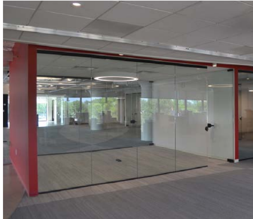
4TH FLOOR TENANT BUILD OUT
