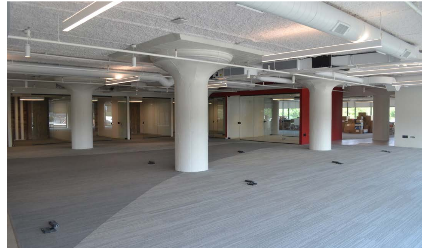
4TH FLOOR TENANT BUILD OUT
