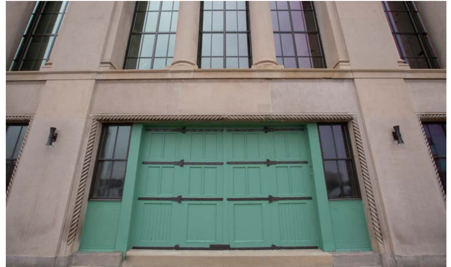
RETAIL A: HISTORIC GARAGE DOOR ON YORK ST.
