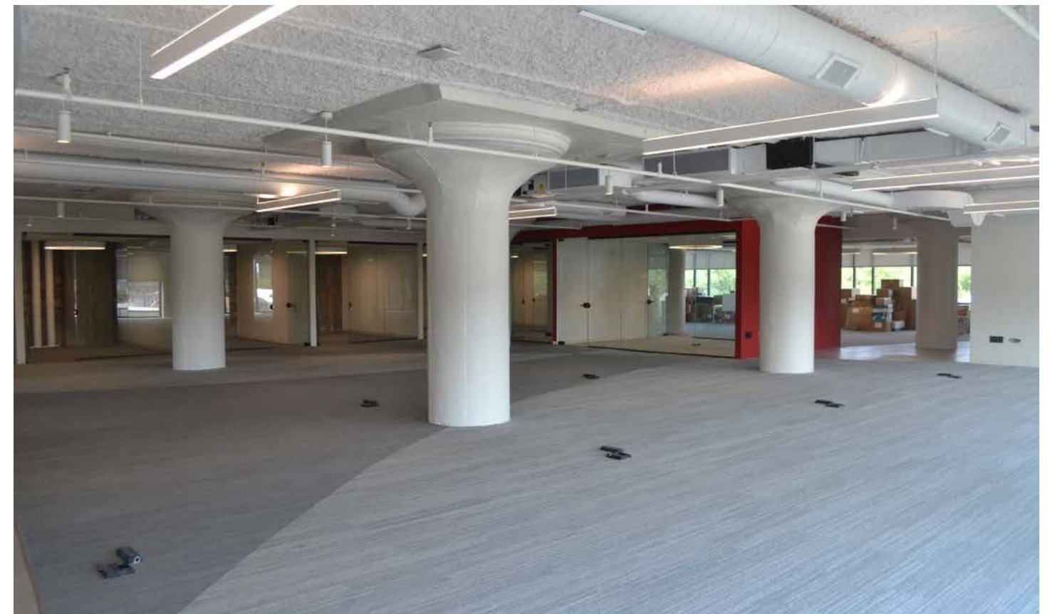
4TH FLOOR TENANT BUILD OUT
